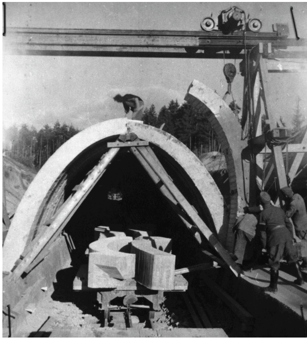
Figure 11: Weingut I, setting the recovery tunnel by precast concrete half-arch segments, 1944, photograph by Polenski&Zöllner(MS a); Figure 12: Weingut I, precast concrete parts for the recovery tunnel; (drawing by students of the University of Applied Sciences, Munich)
