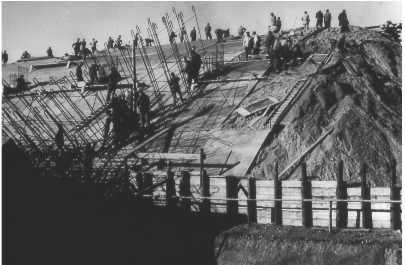
Figure 13: Weingut I, gravel fill for the first arch, 1944, photograph by Polensky&Zöllner; (MS b)
